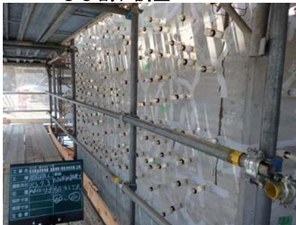
ひび割れ補修
