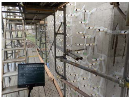
ひび割れ補修
