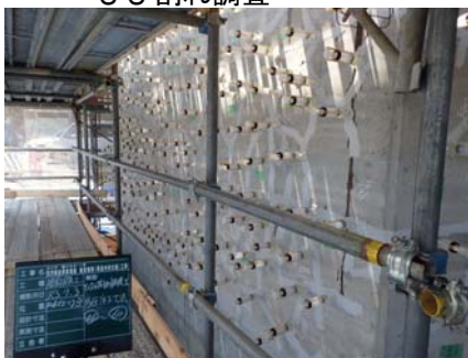
ひび割れ補修
