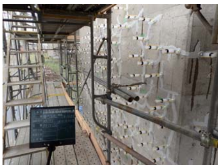
ひび割れ補修
