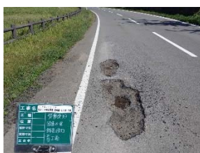
舗装仮復旧前
