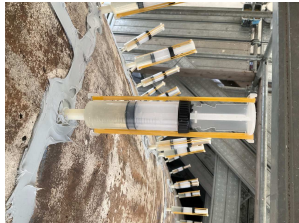
橋梁補修工 ひび割れ補修
